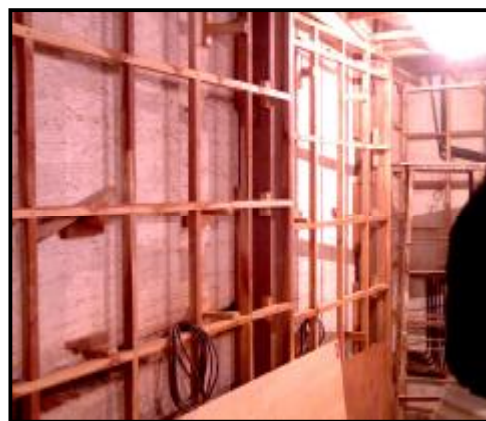
Floating Wall Construction
